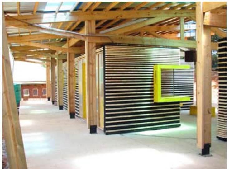
13_Facade Kitchen south
