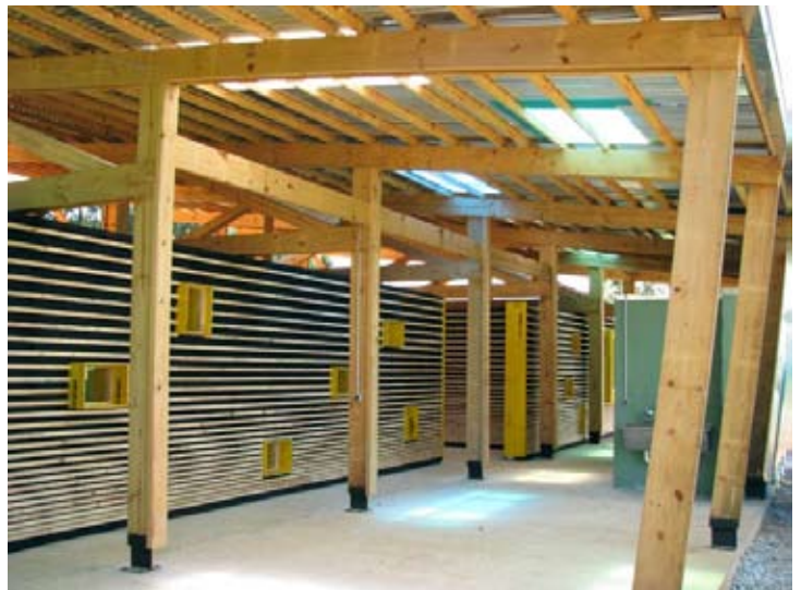
14_Doka-boxes, Preschool Facade south
