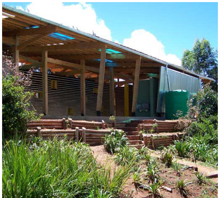
03_South view, approach to building from existing building
